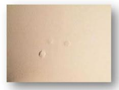
Fastening popping is actually commonly encountered not only in plasterboard but also in timber decking, a variety of wall cladding substrates and long run roofing. "Squeaky Floors" are likely to be a result of fastener popping. This annoying problem has been around as long as we have built with timber framing.
